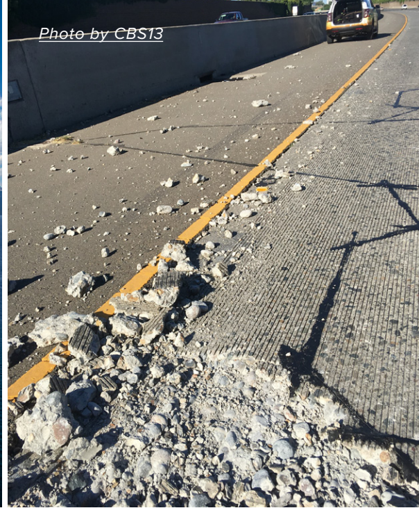
Figure 5: US 50 Pavement Buckling During 2017 Heat Wave
