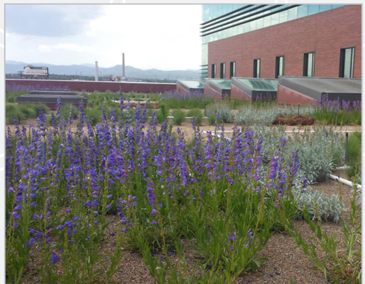
Figure 26: Community College of Denver Green Roof
