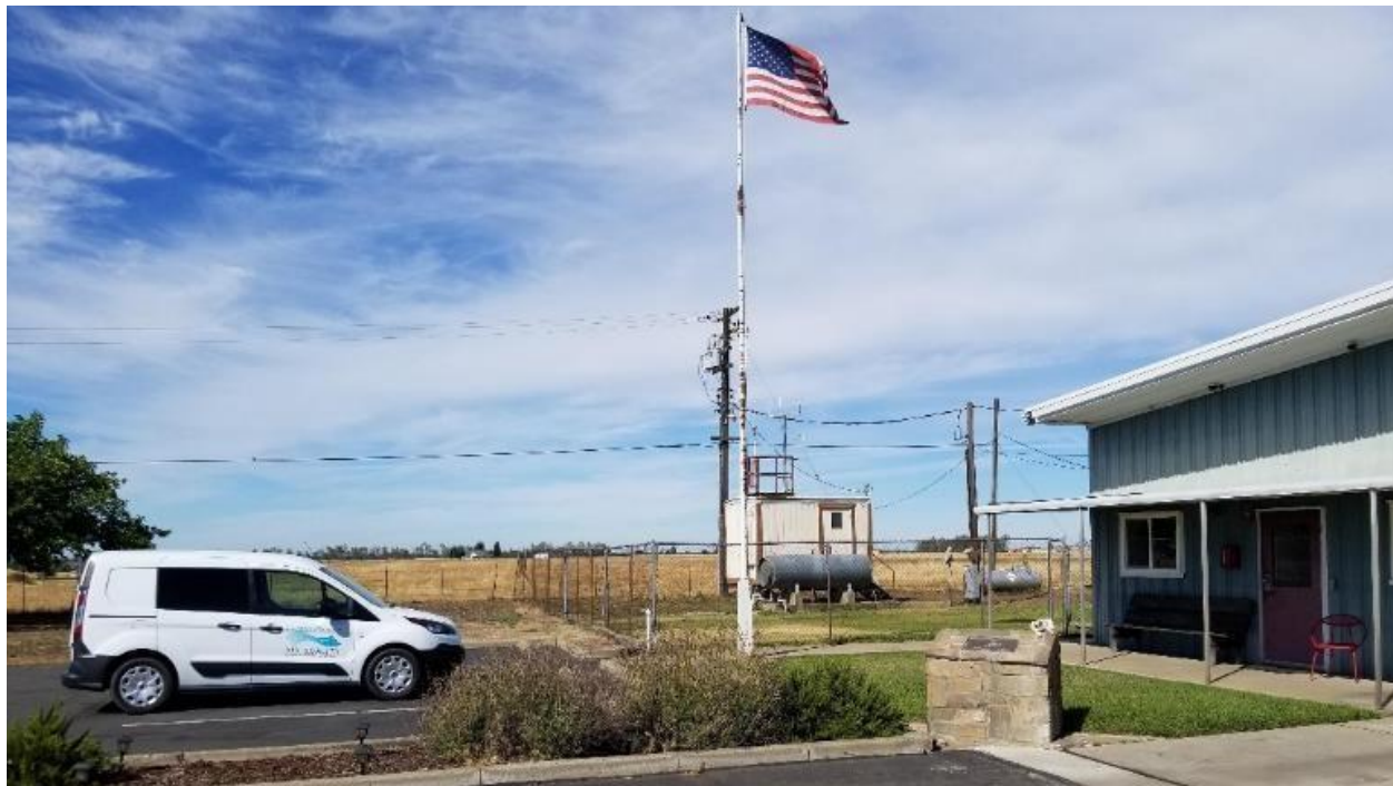
Figure 34 Sloughhouse Site Photo
