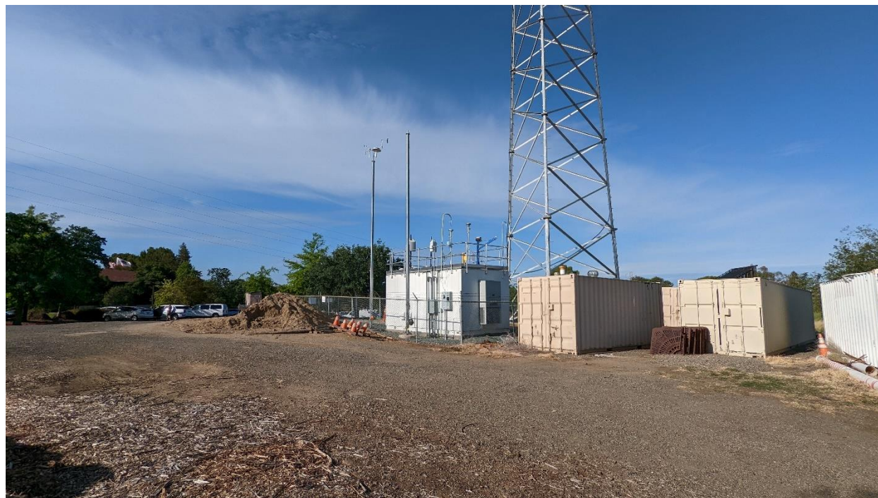
Figure 28 Folsom-Natoma St. Site Photo
