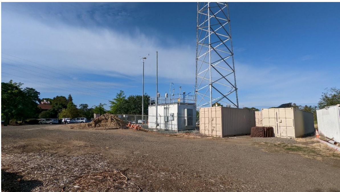
Figure 32 – Folsom-Natoma St. Site Photo
