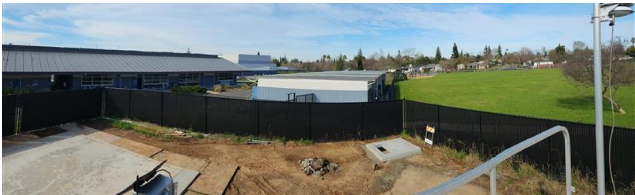
Figure 30 – Panoramic Photo Looking West from Del Paso Manor Temporary Trailer
